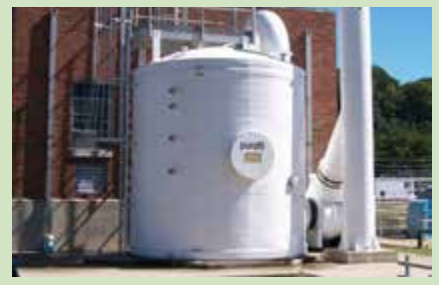
EMERGENCY GAS SCRUBBER Contain catastrophic toxic gas releases Up to 3-ton release or 11,000 CFM
