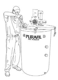
8. Pour the contents of the media sampling probe into the appropriately marked bag. Fill the sample bag to within one inch from its top and seal tightly.
